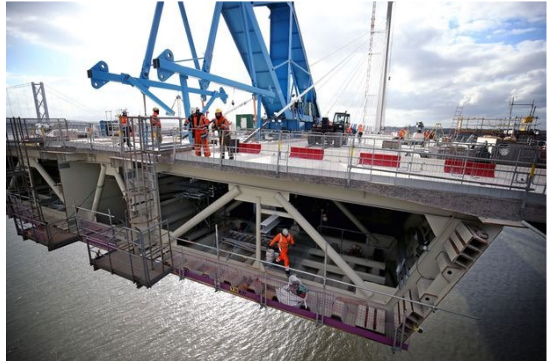
Queensferry Crossing. Ramboll & LAP
